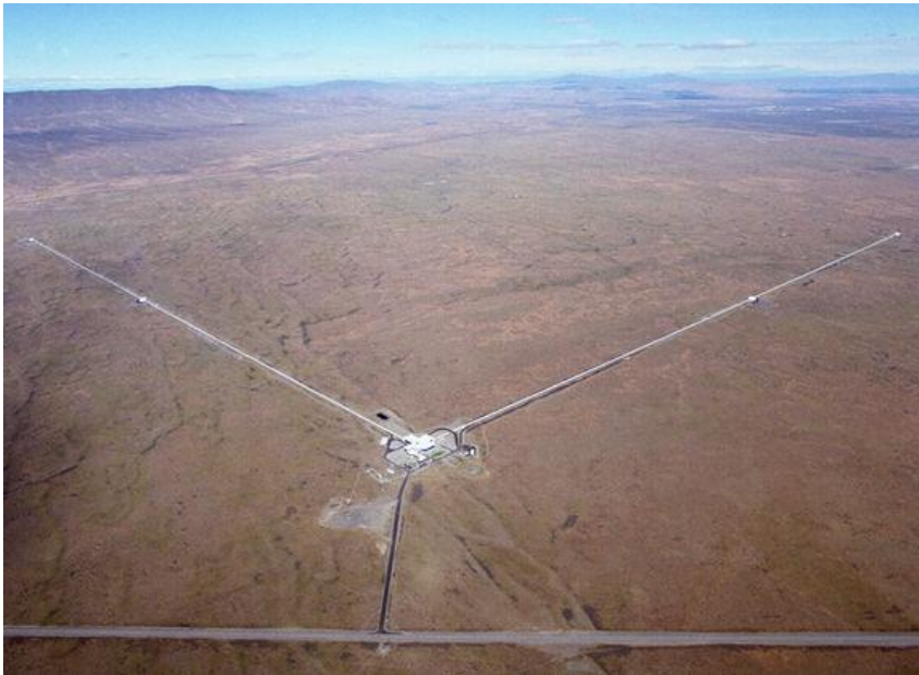
Michelson interferometer \Delta L/L \approx 10^{-22}
